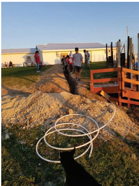
WORK TEAM ASSISTING ON THE CHURCH PROPERTY.
