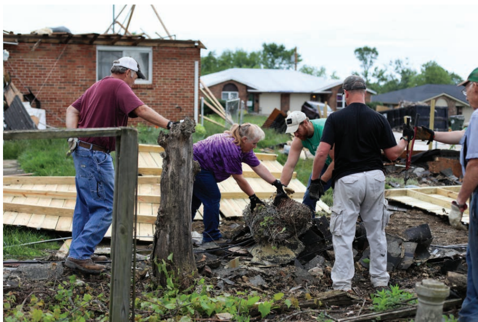
SALEM CHURCH DISASTER RELIEF TEAM REMOVING DEBRIS FROM YARD.
